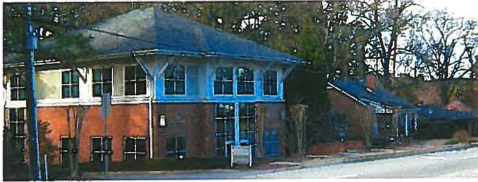
Figure 6-5-8: Similar building materials to adjacent single-family dwellings
