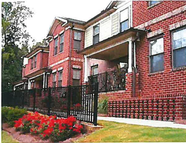
Figure 6-7-4: Facade treatment with covered porches, changes in wall plane, and distinct changes in color and texture
